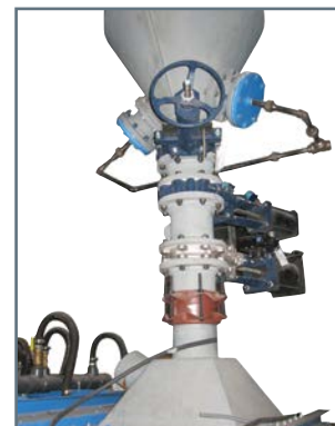
Knife gate valve inlet arrangement
