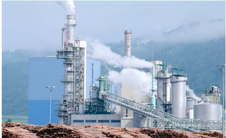
With more than 350 units, B&W has the largest installed base of recovery boilers in the world.
