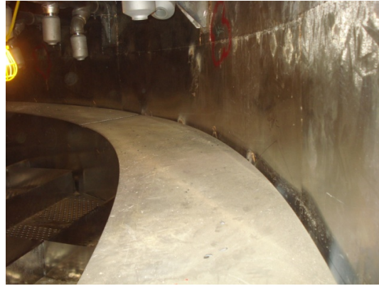
Figure 1 – Typical wall ring retrofit in a wet FGD
